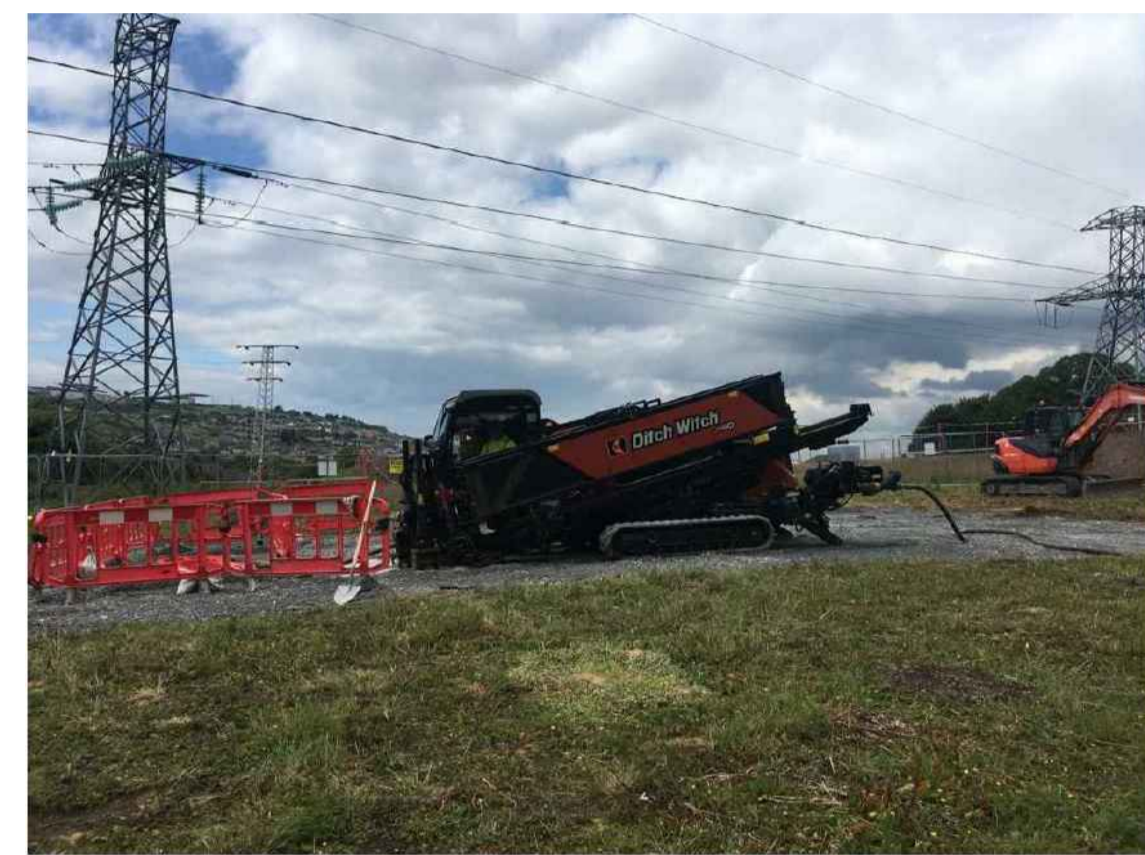
Image 1 : Typical Directional Drilling Rig
